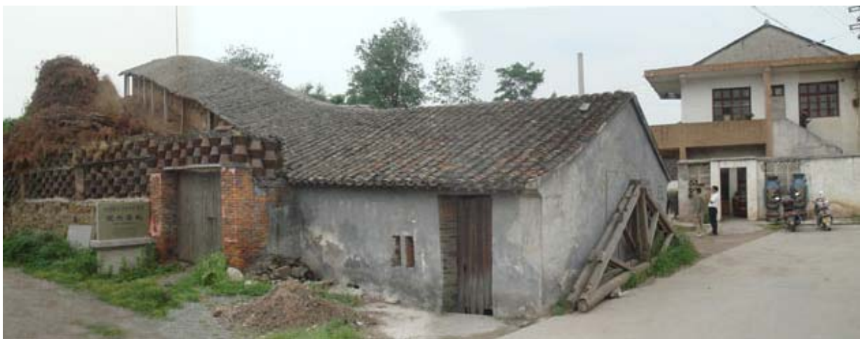
Dragonkiln (long furnace) in Yixing. The small building down below is the fireplace. Going up the artificial hill is the kiln made of clay were the ceramics are fired. The chimney is uphill. The rooftiles keep the kiln from wetness. This is the last remaining kiln left in the area, it is believed to be 300 years old. For preheating and firing, that takes 38 hours, 5000 kg of dry pinewood is used. Before World War II there used to be ten of these enormous kilns in this area. Photo Jeroen Bechtold.
